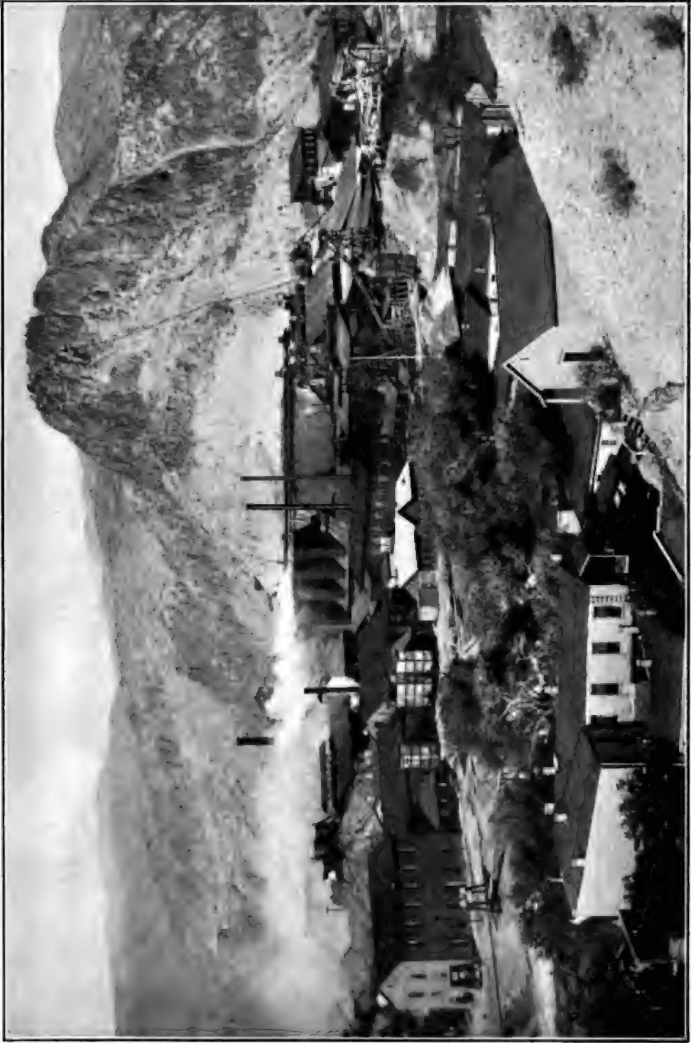
The great reduction works are far below the mines, and by inclines, tramways, chutes, and steam-cars the ore steadily goes down • • • until it is at the smelter
